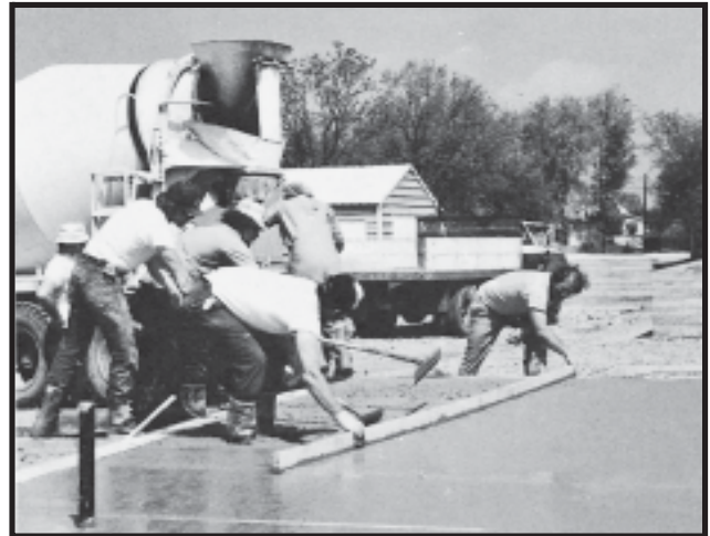
Finishing Concrete Flatwork
